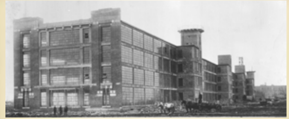
Ford Highland Park Plant, Building A under construction, 1909
