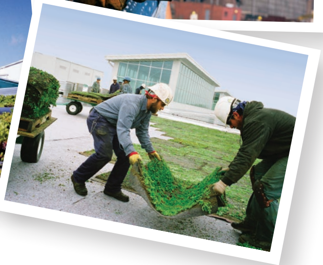
Left: The sedum roof of the Dearborn Truck Plant. Bottom right: Workers planting the roof. Top right: Worker with the famed Rouge smokestacks in the background.
